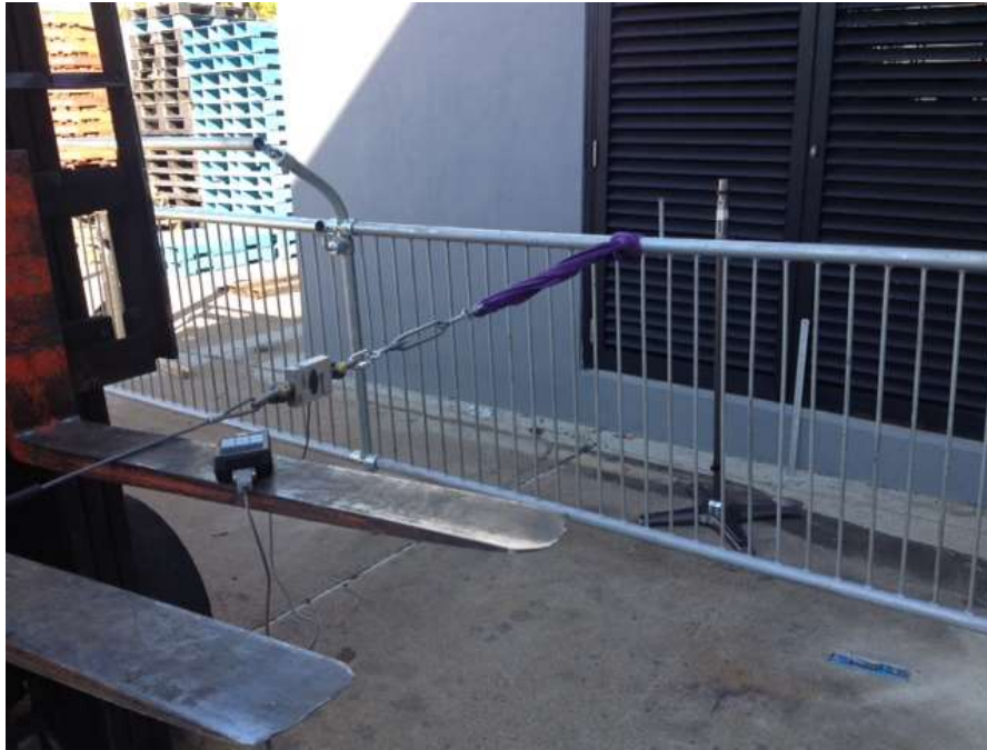
Photo 1: Test # 2 Pedestrian Panel 2.4mts Top rail
