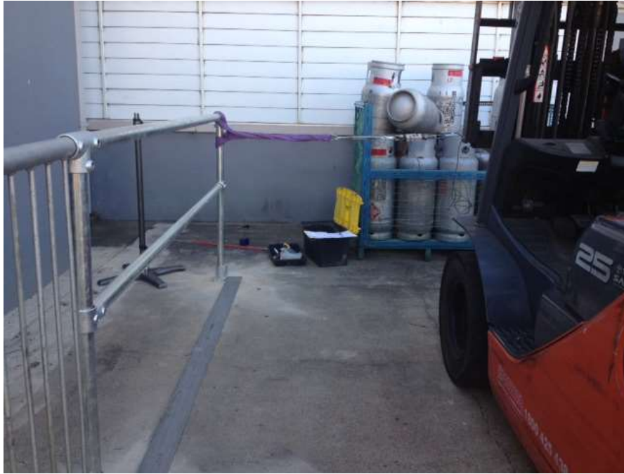
Photo 1: Test # 1 Handrail 2.4mts Post
