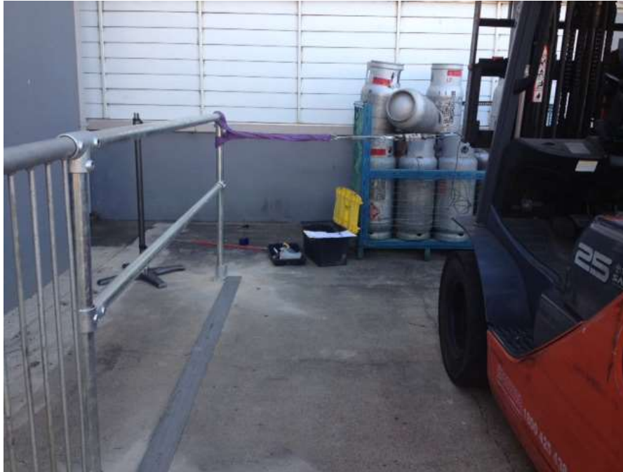
Photo 1: Test # 1 Handrail 2.4mts Post
